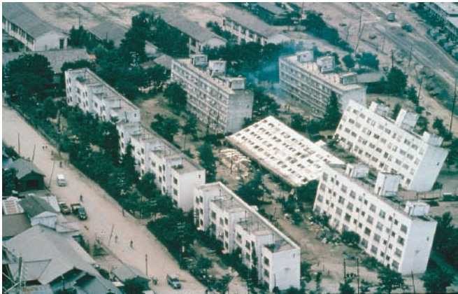
(A) Earthquake of June 16, 1964, Niigata, Japan. Apartment houses tilted by liquefaction. About one-third of the city subsided as much as 2 m as a result of sand compaction. (Courtesy of U.S. Geological Survey)
