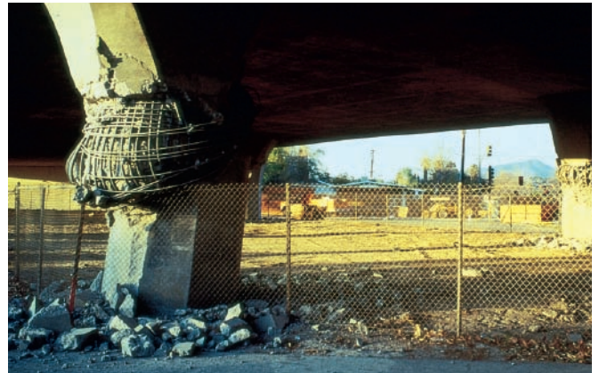
(B) Earthquake of January 1994, Northridge, California. Extensive damage to freeway overpasses occurred. (Photograph by Geo-Tech Imagery)
