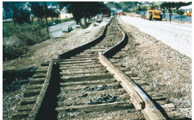
(D) Earthquake of February 9, 1971, San Fernando, California. Southern Pacific railroad tracks near Los Angeles were laterally displaced. (Courtesy of U.S. Geological Survey)
