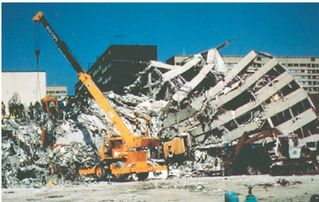
(C) Earthquake of September 19, 1985, Mexico City, Mexico. A 15-story reinforced concrete building collapsed. (Courtesy of U.S. Geological Survey)
